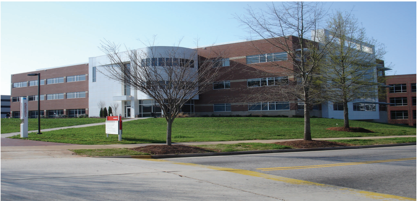
Partners III GSF 82,988 Cost $22,320,211 Designer: Freelon Group Contractor: Shelco, Inc. MBE Participation: 26.8%
