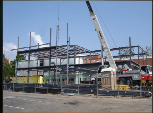
Student Health Center - Addition
