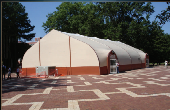
Atrium Food Court Renovation – Phase 1
