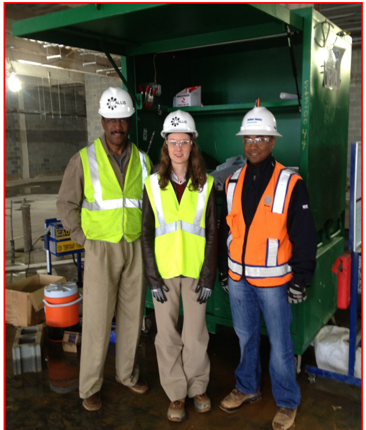
(Left to right) Jesse Callis - Callis Construction, Rachel Allen—Callis Construction and Donovan Everett—Balfour Beatty Construction.
