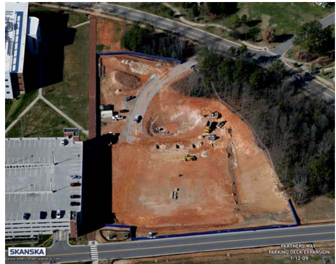
Partners Way Parking Deck Expansion—Skanska/H. Richardson Co. 4 Level Deck—400 Spaces Cost $5,069,000 MBE Participation 35.35%
