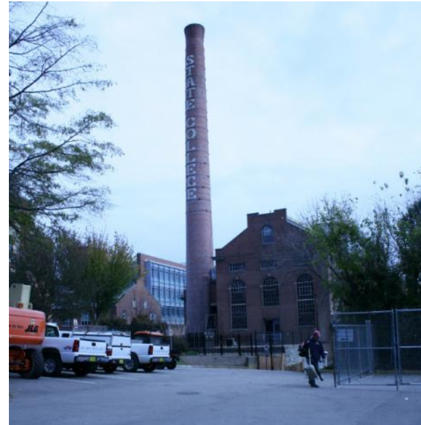
Photo 24: View of Yarbrough Plant, electrical switch gear just in front of old building. Service vehicles stored in parking area to left
