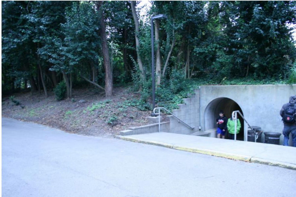
Photo 10: View of grade change at East Tunnel
