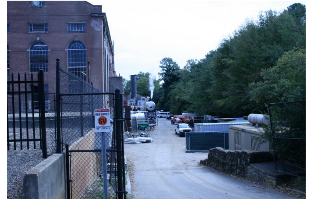
Photo 25: View access ramp from parking area to service yard along south face of Yarbrough Plant
