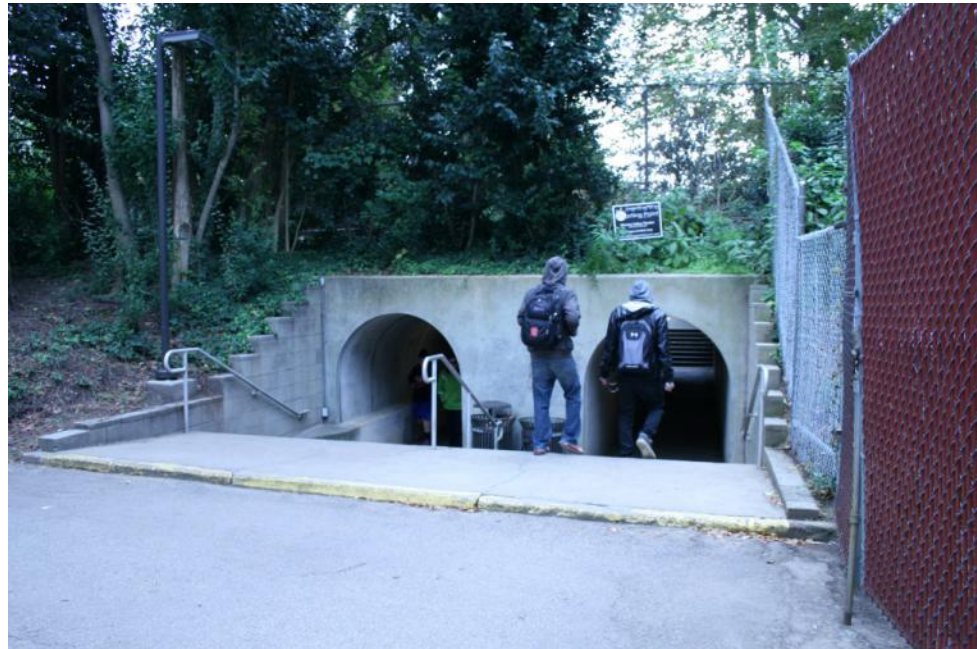
Photo 27: View of East Tunnel, rail road above asphalt in foreground.
