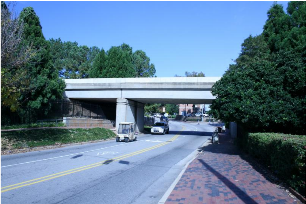
Photo 16: View of Dan Allen Drive, looking north towards Yarbrough Drive
