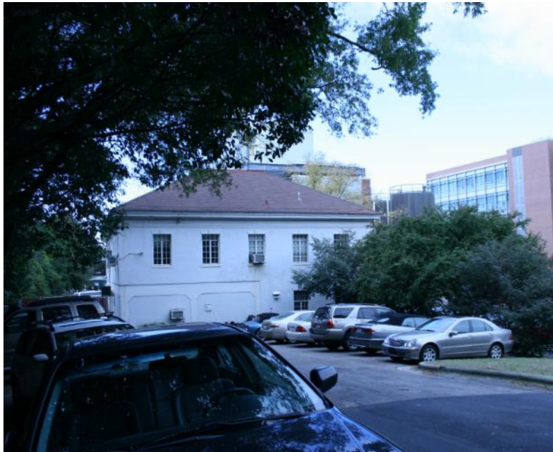
Photo 26: View of parking area east of existing field house, North Deck parking project will remove this parking. Field house is approved for demolition 2013 calendar year.
