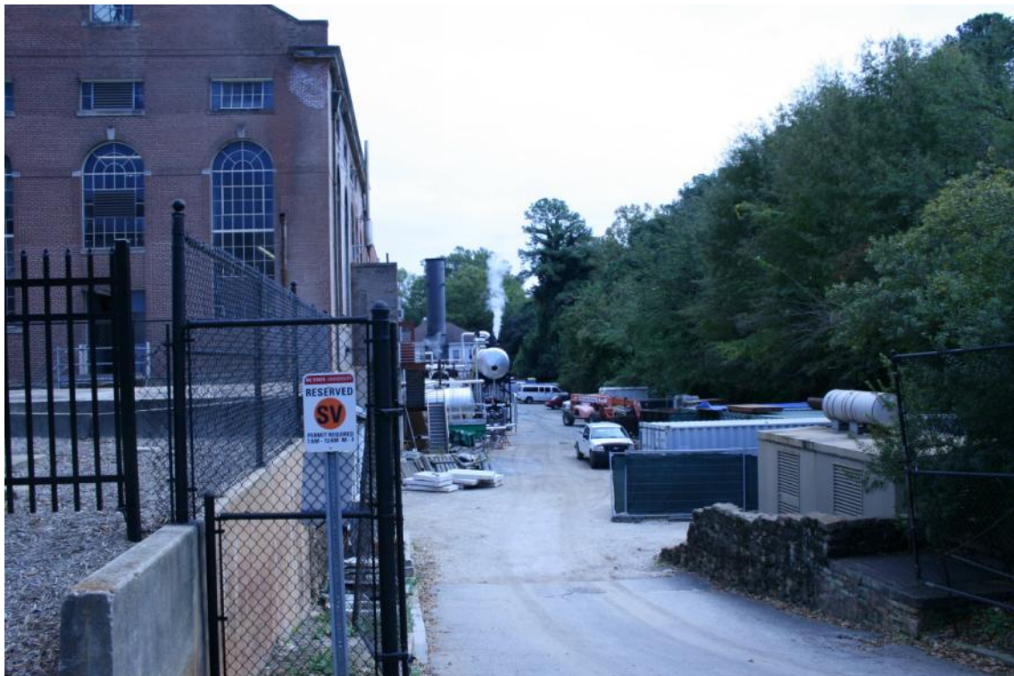
Photo 13: View of access drive at south of Yarbrough Plant
