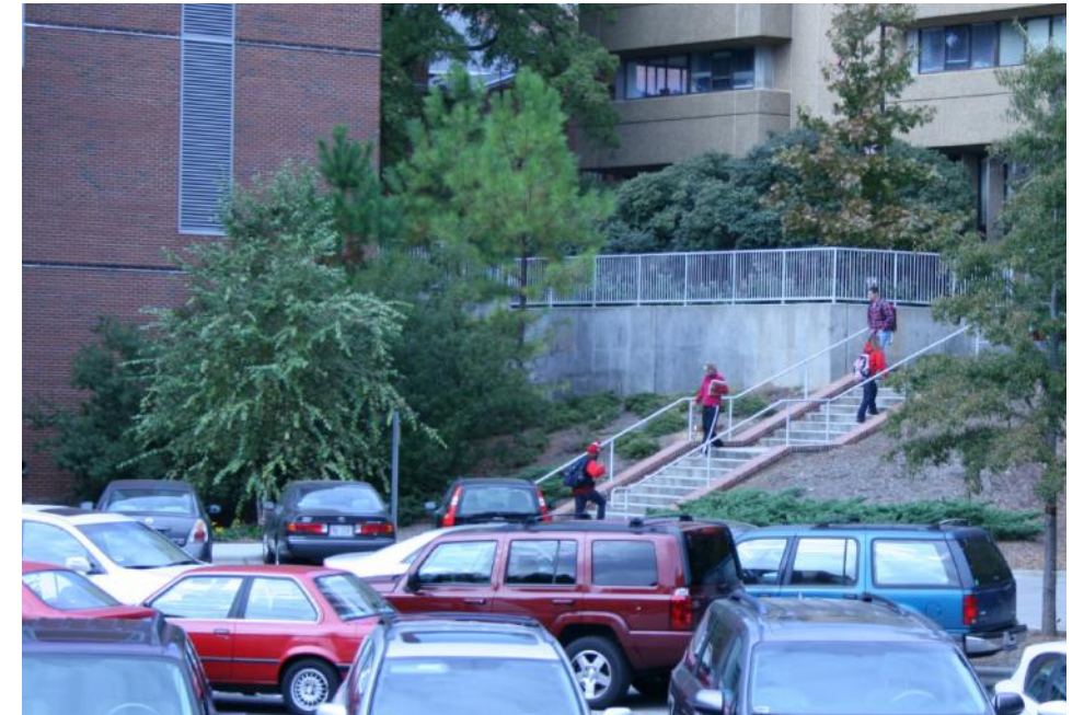
Photo 12: View of stairs at the pedestrian walk leading to Stinson Drive, taken from Boney Parking Lot
