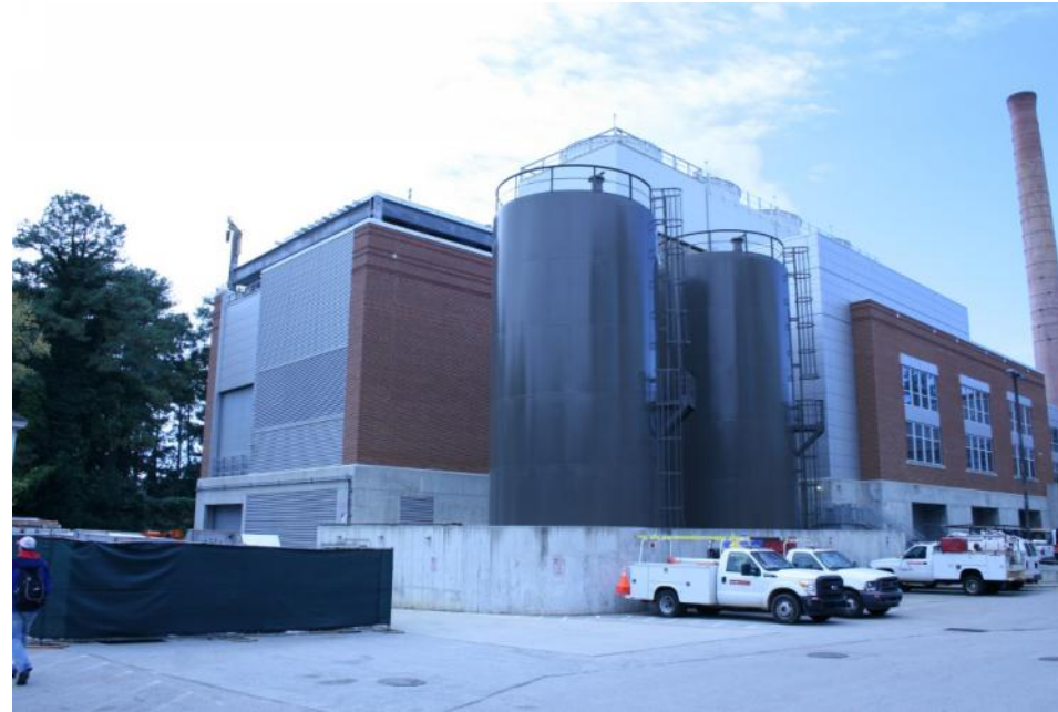
Photo 11: View of oil fill point at east side of Yarbrough Plant
