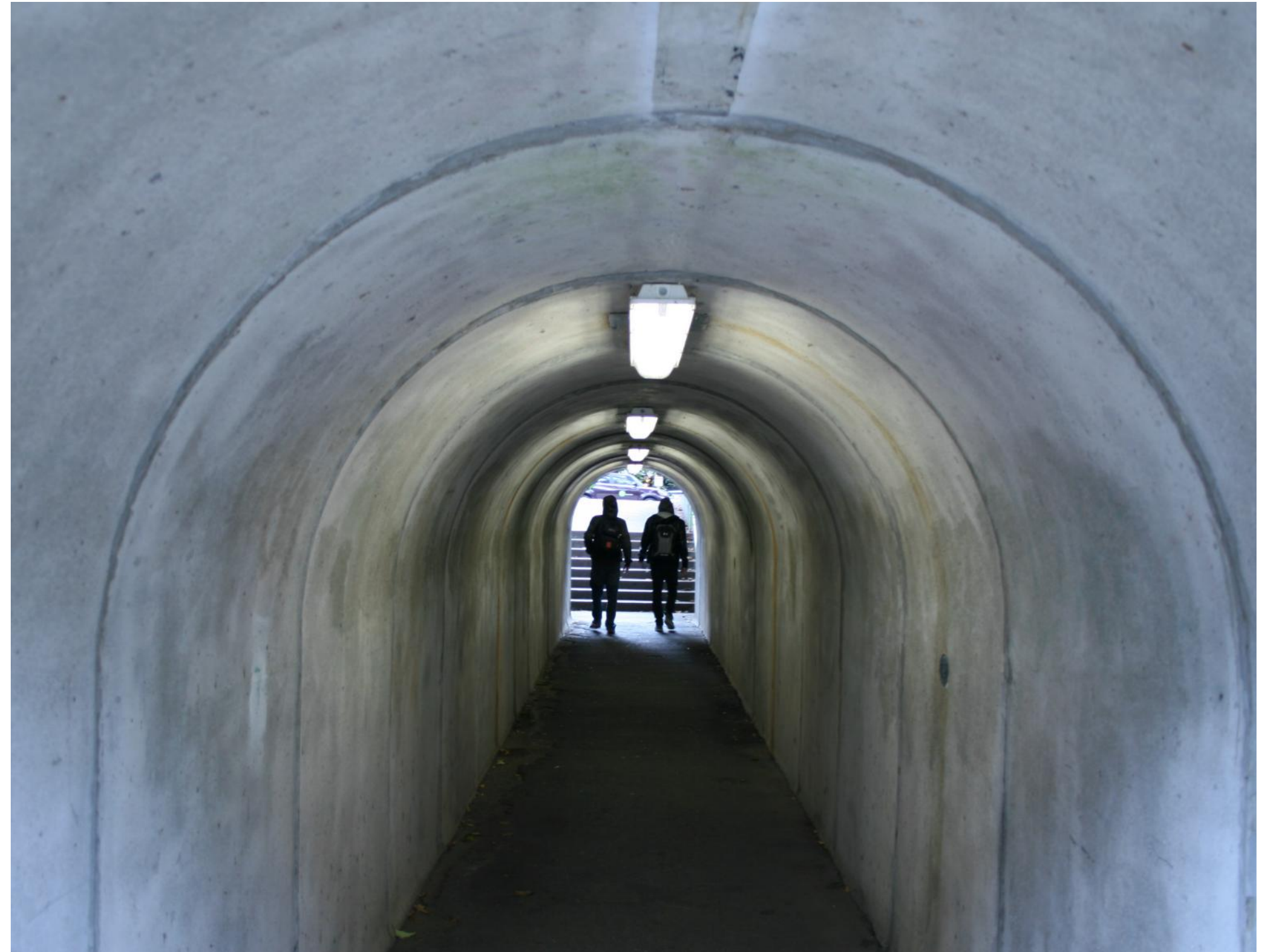
Photo 9: View of East Tunnel looking south
