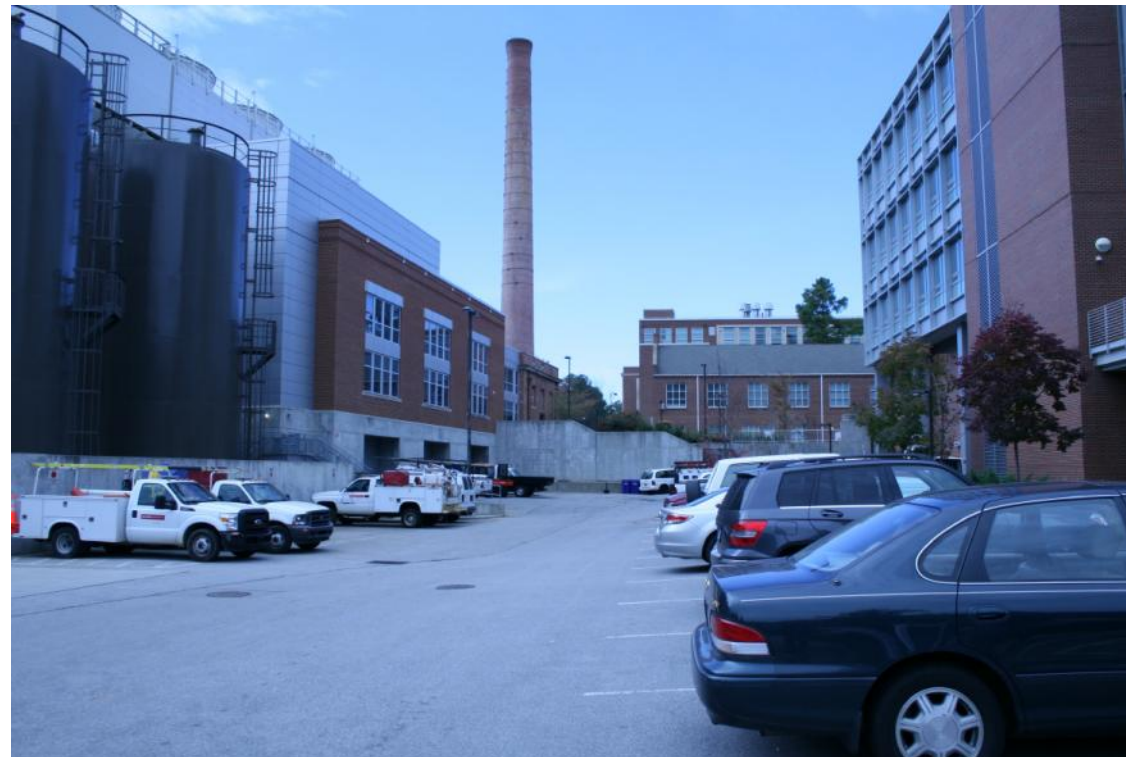
Photo 14: View of service yard at Yarbrough Plant
