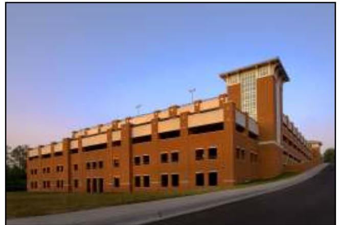
Parking Deck G at UNC-Charlotte
