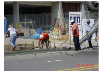
H. Richardson and company at work on Schaub Hall.
