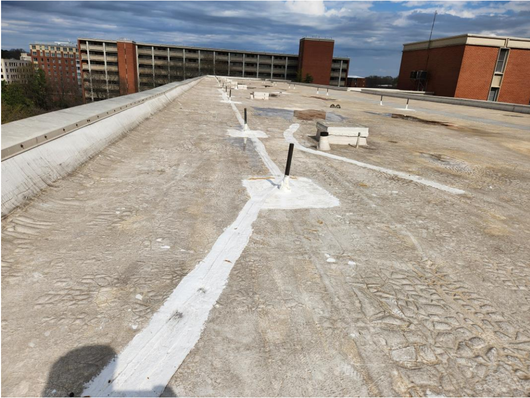
Roof at Lee Residence Hall
