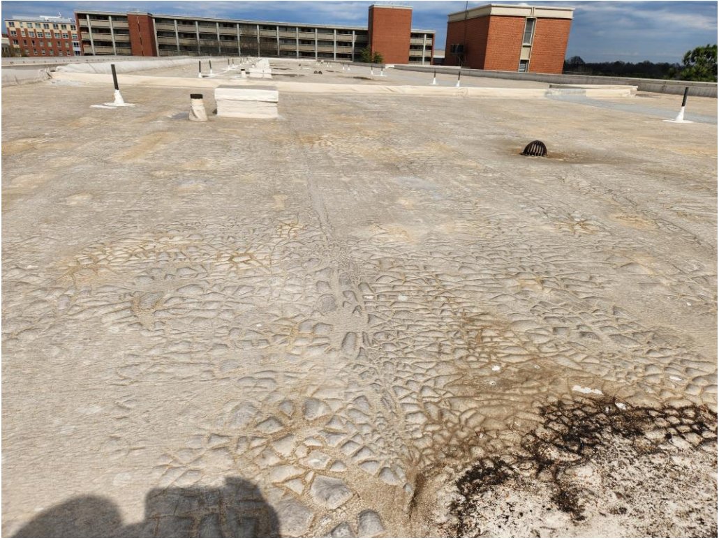
Roof at Lee Residence Hall
